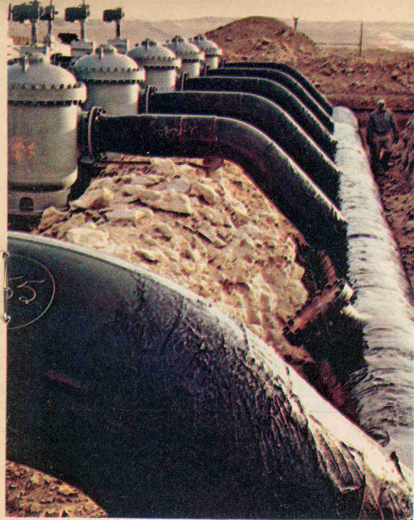
LEFT — pipeline for Continental Oil Company crosses miles of barren Middle East desert.
